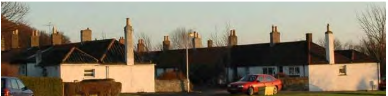
The chimneys are an important element of the view towards Double Row.
