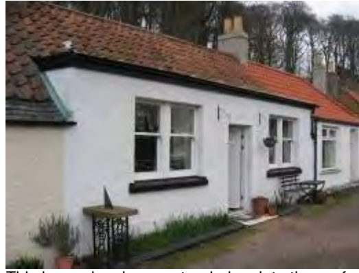
This house has been extended up into the roofspace and the window openings heightened.
