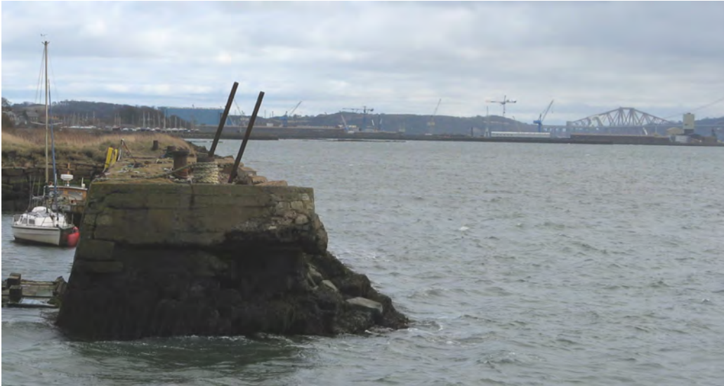
View to the east, with the Forth Rail Bridge and Rosyth in the background.
