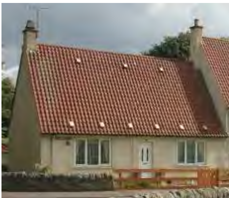
Single storey house at the Cairns
