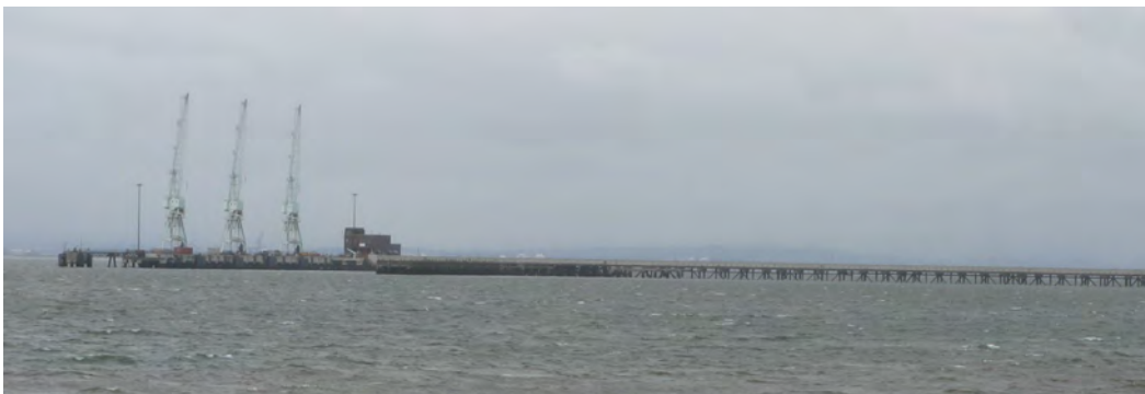
View west from Charlestown Harbour, to Crombie Pier
