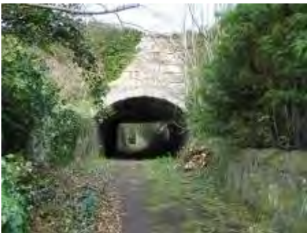
View north along the cutting
