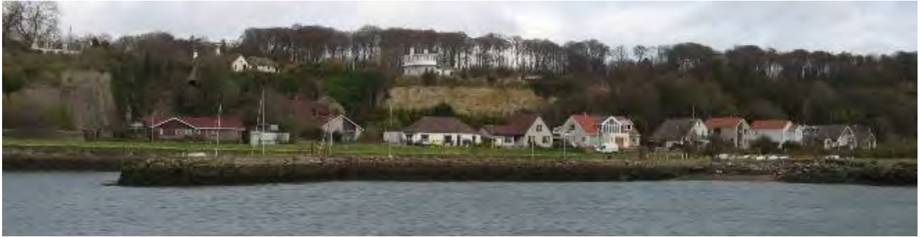
The housing at East Harbour Road seen from the west outer pier
