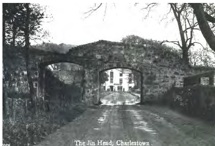
The Gin Head bridge c.1900, central part now demolished, but abutments still visible. (Simpson & Robertson)
