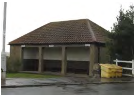
The shelter and public toilets on Main Road
