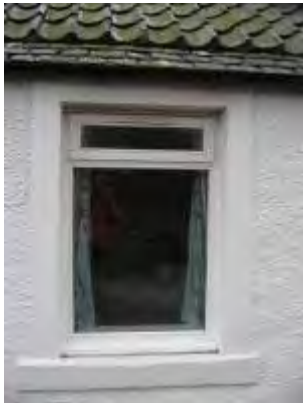
A range of inappropriate replacement windows, not matching original opening sizes, materials or design.
