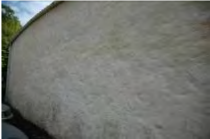
The Scottish Lime Centre: north-east wall
