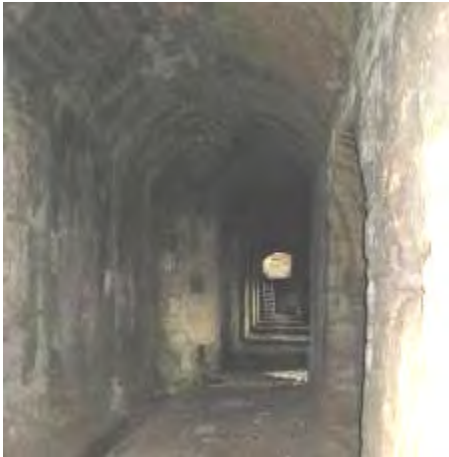
View of the interconnecting passage at the back of the kilns
