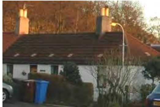
Roof ventilators in a pantile roof
