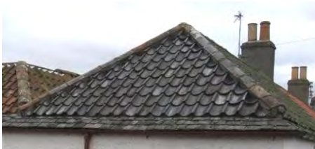
Black glazed clay pantiles with slate easing on South Row
