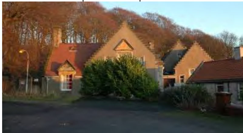
The west (principal) elevation of the Queen's Hall
