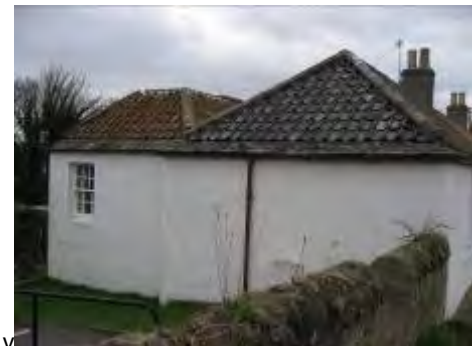
An extension on South Row
