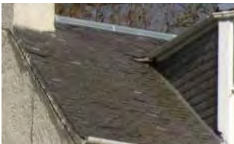
The Old Inn, south roof pitch
